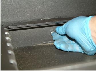
It is necessary to add further loose fill around the flue liner at the top of the Cassette Box, particularly on external chimney situations. The liner may need shaking to help loose fill fall completely down to the stove.
